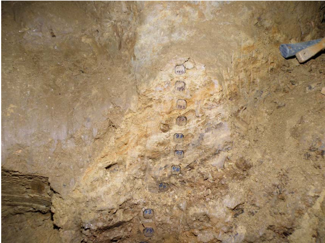
Photo 5 Segment HH74 to HH110
